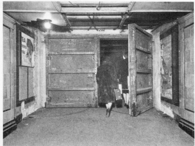
Flood doors fitted to station entrances and subways
